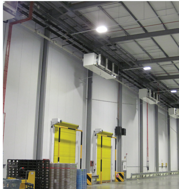
Loading area separated from processing area by vestibule. This acts like an air chamber, reducing the ingress of warm air to temperature controlled areas.
