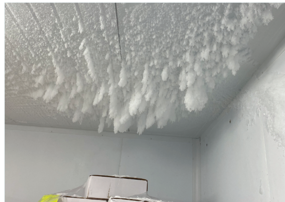
Ice build-up indicates issues with ceiling insulation or door seals.
