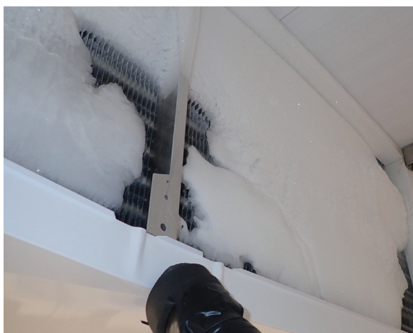
An example of poor maintenance of the evaporator coil: ice builds up on the evaporator coil, which reduces air circulation. In this case, check the expansion valve and the defrost set up.
