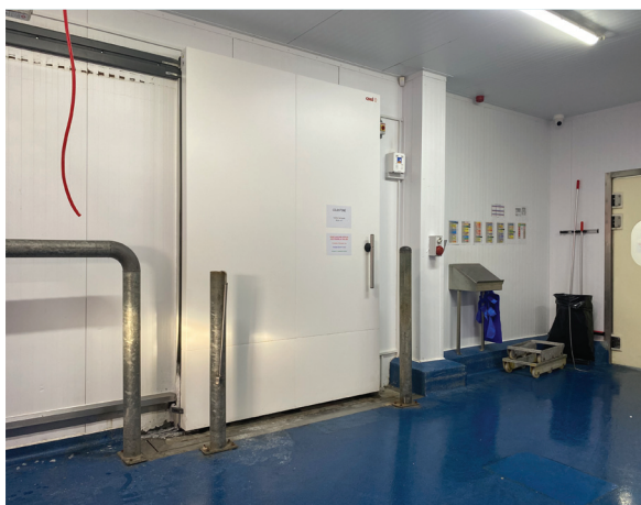
An example of good protection for cold room door openings.
