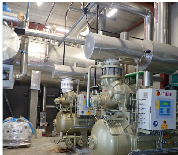
A well maintained plant room showing compressors and refrigerant vessels.
