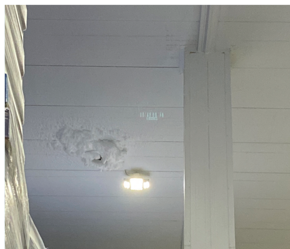
Ice build-up on the pressure relief valve limits the airflow to the valve.
