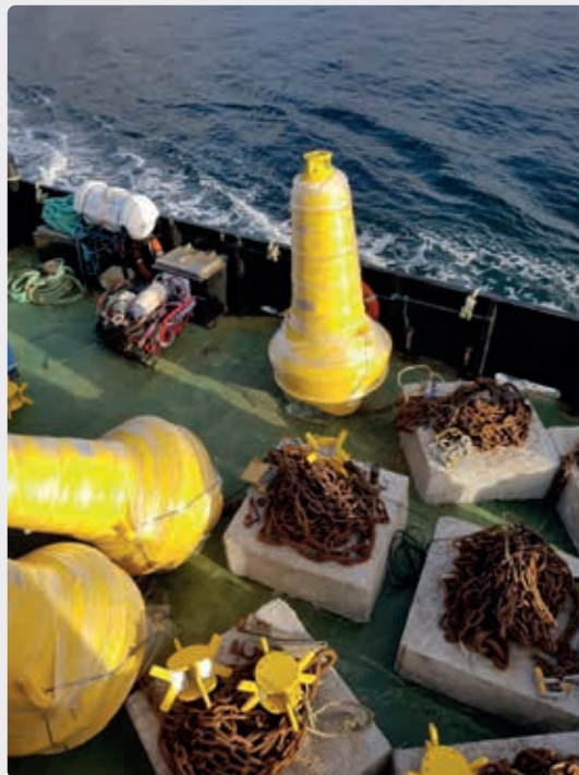
Figure 1: Mooring equipment being brought to site.
